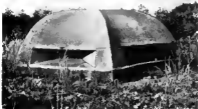
Figure 15. Here is a decoy pillbox constructed of wood, covered with burlap or ornburg, and sprayed with paint to resemble concrete. Sand and dirt may be sprinkled on the wet paint to give it a concrete-like texture.
